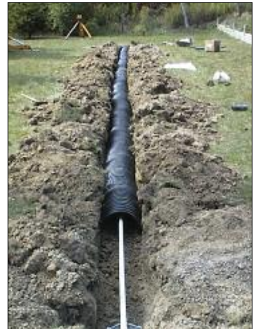
Single line shallow buried trench.
