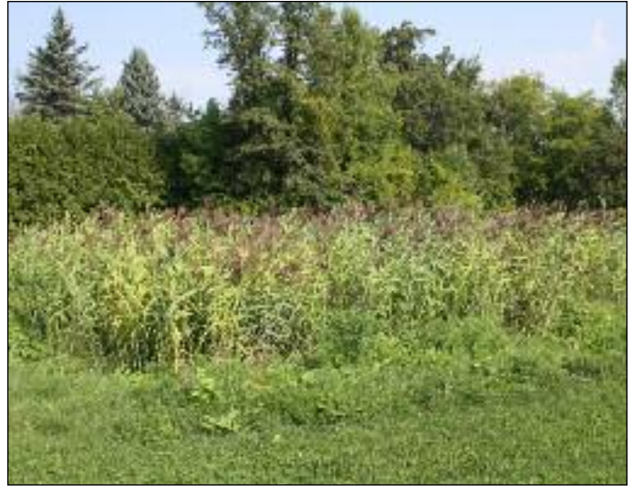
Subsurface constructed wetland.
