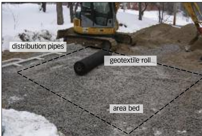
An area bed showing stone layer, pipes and geotextile fabric.
